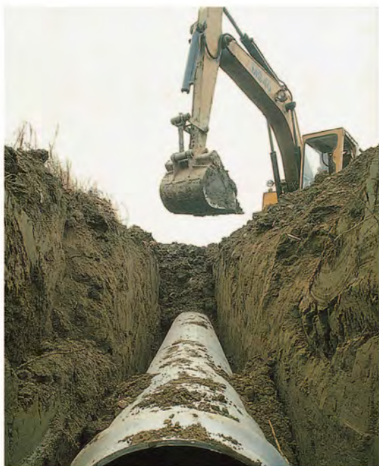
▲自来水工程 Water supply engineering
