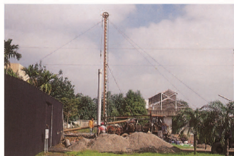
▲ 凿井工程 Well drilling engineering
